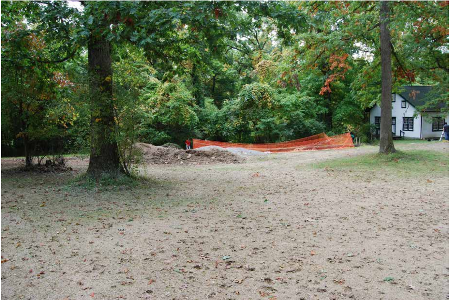
PHOTO | View of site facing southwest (Phase I construction)
