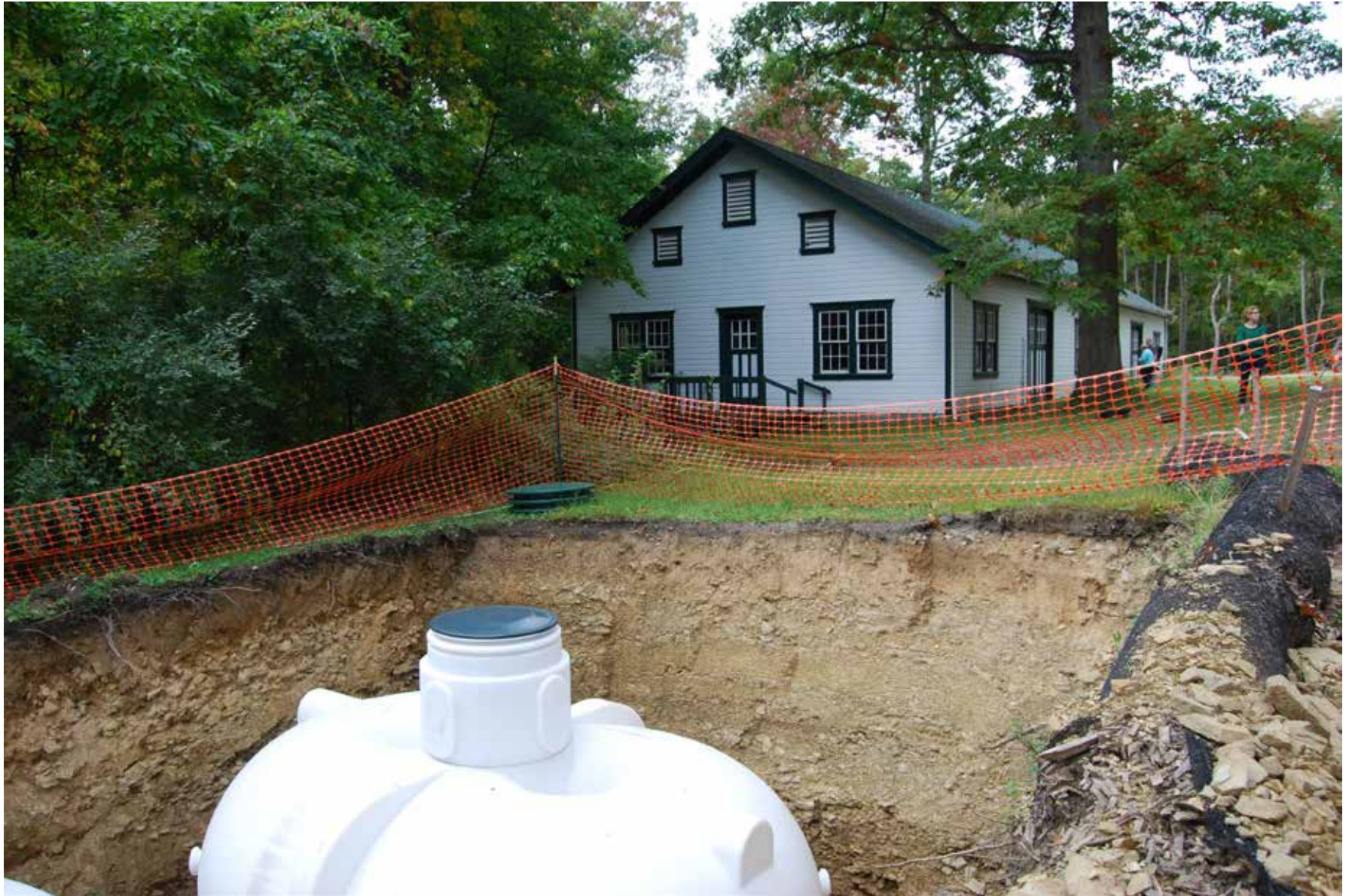
PHOTO | View of site facing west (Phase I construction)
