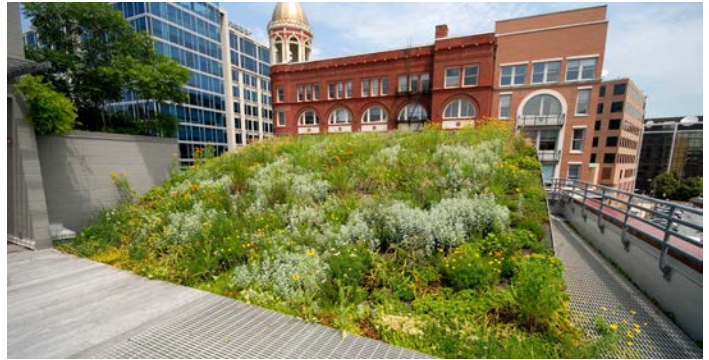
ASLA headquarters' green roof is one example of how landscape architects help reduce stormwater runoff while also conserving energy and improving air quality. Firm: Michael Van Valkenburgh Associates and Conservation Design Forum. Photo: ASLA
