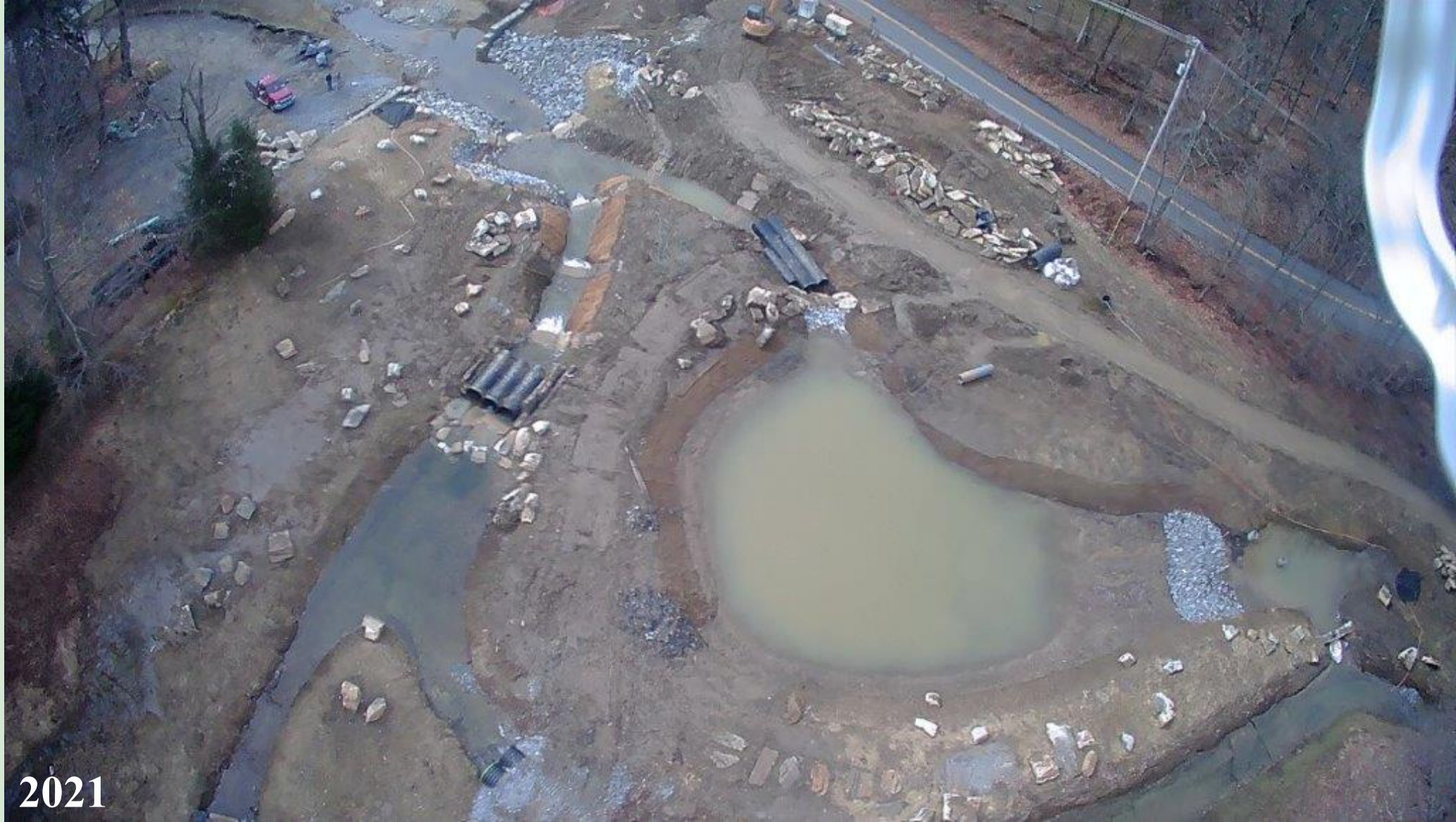
Drone photograph of the park under construction with dam wall remnant at upper left. Pond in center with forebay to the right. A weir below the forebay spins water into the pond in controlled manner from the primary stream reach in the lower right.
